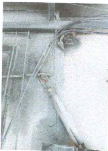
BURNT MAIN BREAKERS AND ELECTRICAL WIRES
